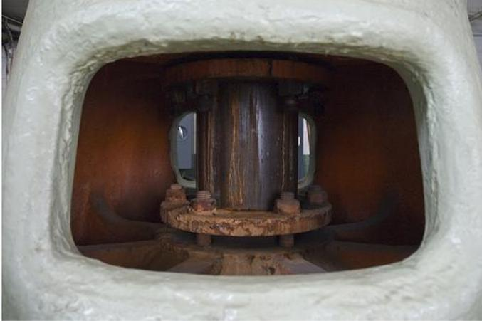
Fig 4. Piston that controls water flow at the end of the penstock at Boulder Canyon Hydroelectric facility.
