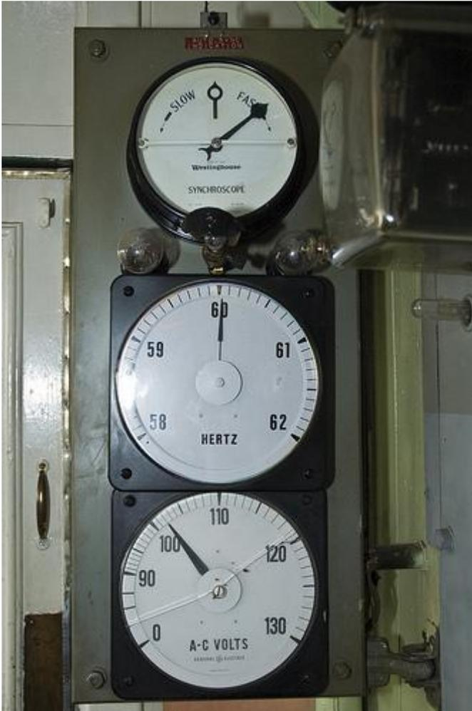
Fig 2. Control panel showing the synchroscope (top), hertz meter (middle), and voltage meter (bottom) at the Boulder Canyon Hydroelectric facility.
