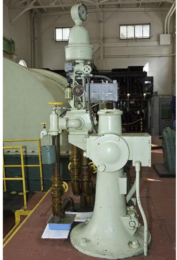
Fig 3. Synchroscope for generator "B" at Boulder Canyon Hydroelectric facility.
