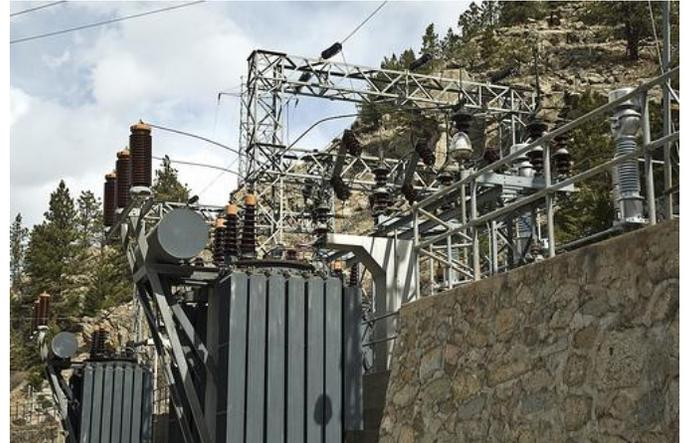
Fig 6. Switchyard next to Boulder Canyon Hydroelectric. The two 12.5 kVA; 115kV Wye/ 4kV Delta transformers can be seen near the bottom left quadrant.
